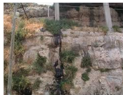
Photo 6.18: Leakage of wastewater from the cesspits in Battir city
