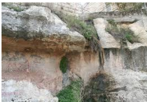
Photo 6.18: Leakage of wastewater from the cesspits in Battir city
